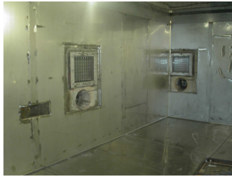
Figure 10: Washing cell picture with portholes and water injection systems
